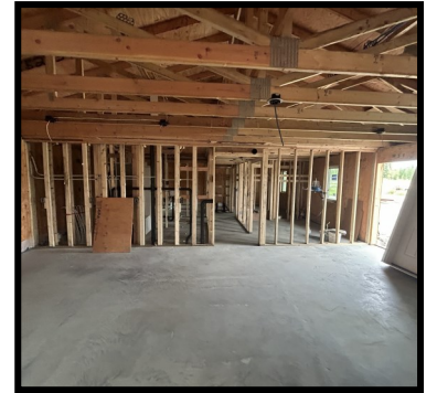
Below Pictures: New Construction in Mendone Subdivision
