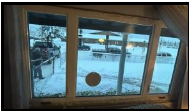
Below: New Window replacement.
