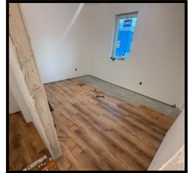
Below Pictures: IRHA Construction Staff rehabilitating a house
