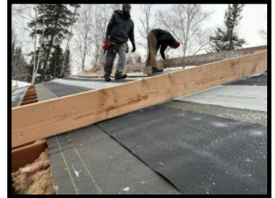
IRHA Staff rehabilitating a roof.
