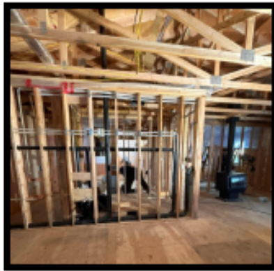
Inside view of the Huslia House re-build
