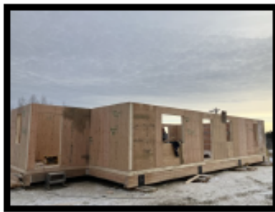
Putting up the frame
