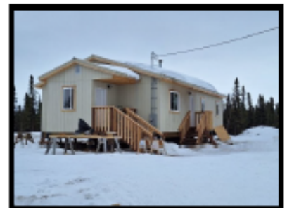
Outside view of the Huslia House rebuild
