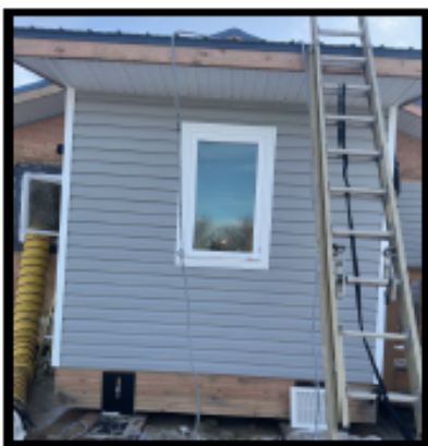
Huslia fire rebuild
