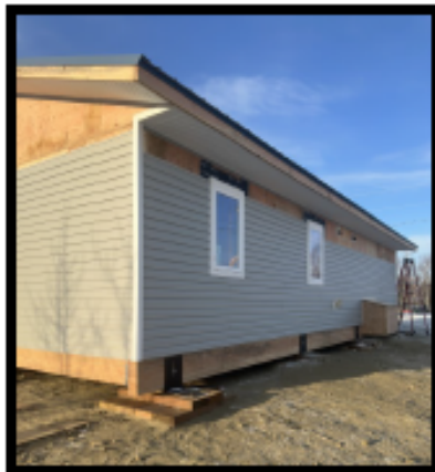
Huslia fire rebuild
