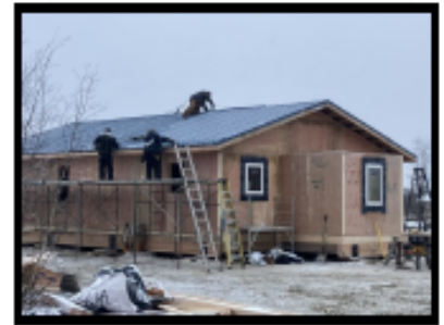
Outside view of the Huslia House rebuild
