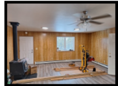
Inside view of the Huslia House rebuild
