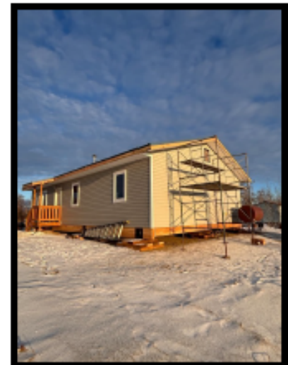
Putting up siding on the Huslia House rebuild
