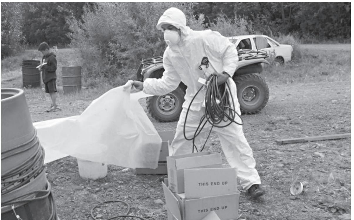
*In Rampart, a weatherization crew member prepares to apply spray cellulose in the attic of a village home. In order to minimize contact with the material, workers "suit up", use breathing masks and follow other safety guidelines.*
